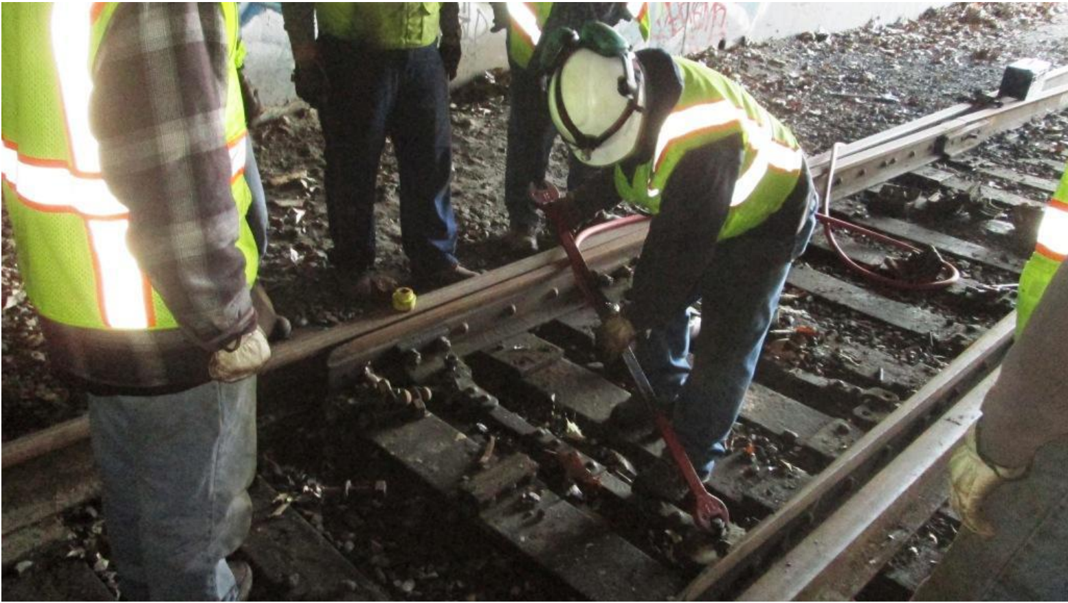
Joe begins removing a connecting-rod by unbolting it from the transit-clip
