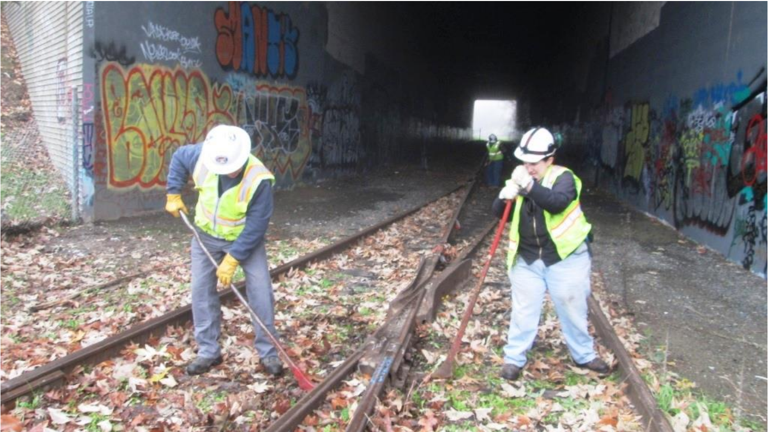
Ed M. and Heather pull spikes at the Setzer switch frog
