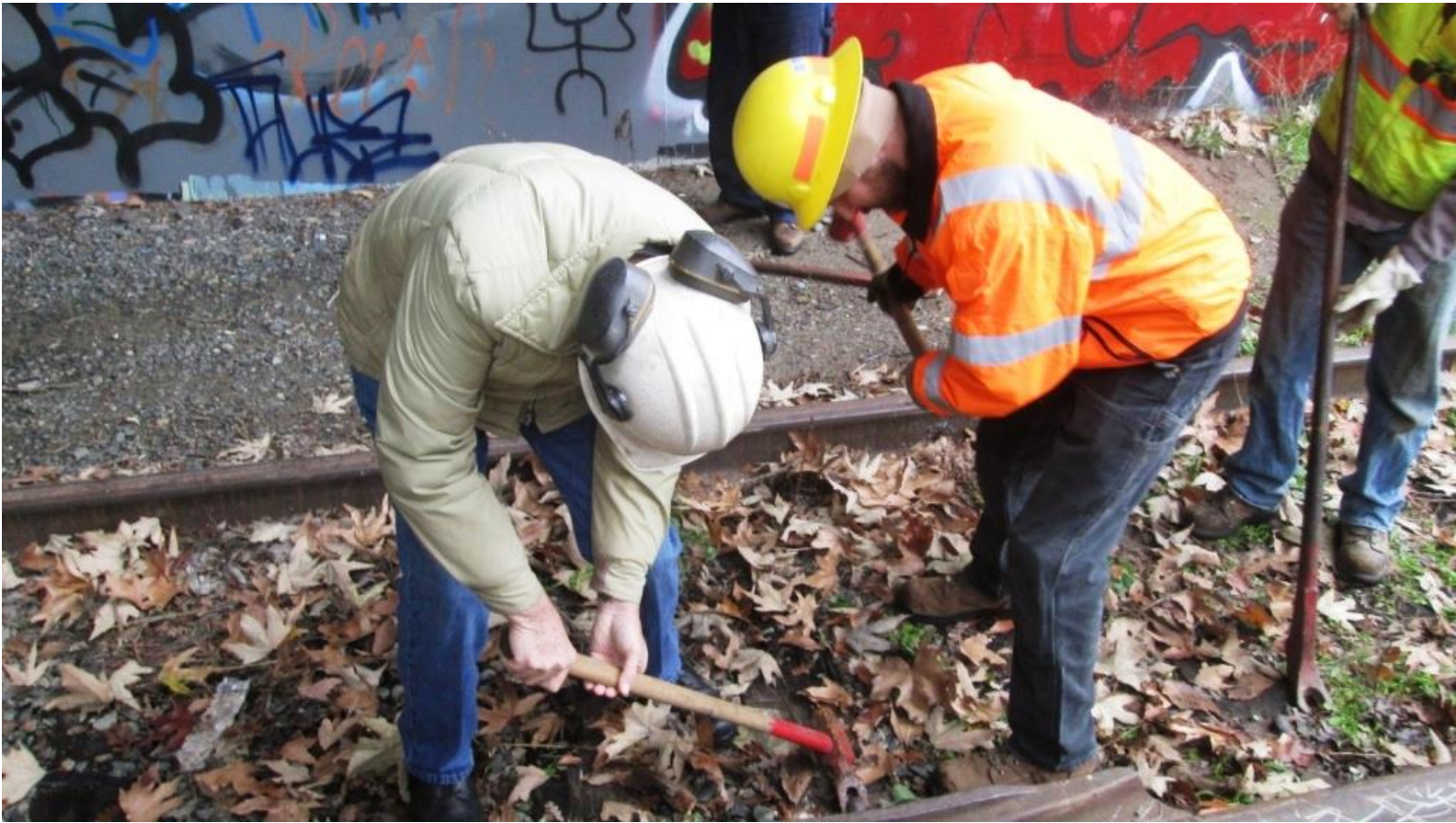
Chris M. employs the sledgehammer to drive the spike lifter, which Alan is holding, under the head of a spike
