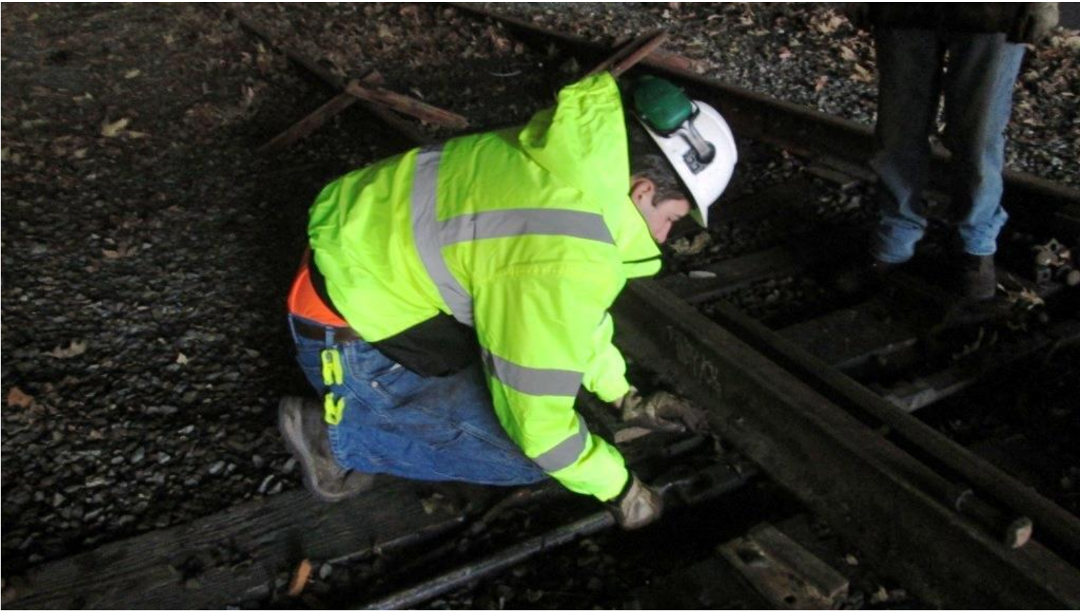
Now Weston pulls the other end of the switch-rod from the connecting-rod
