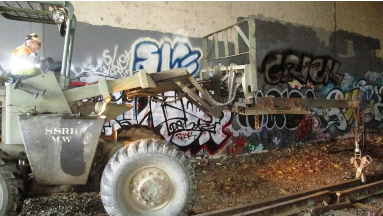
Cue Mike F. on Big Green to lift the rails in an attempt to separate them from the ties
