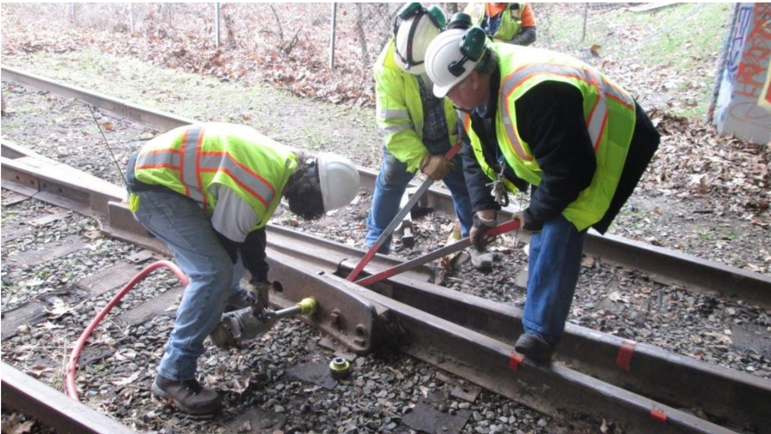
Frank and Chris C. apply pressure to a bolt with track wrenches to stop it from spinning as Matt uses the impact wrench to remove the nut
