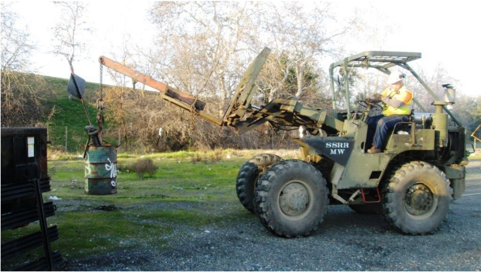
Mike F. loads a barrel containing switch components and the switch-stand onto the truck
