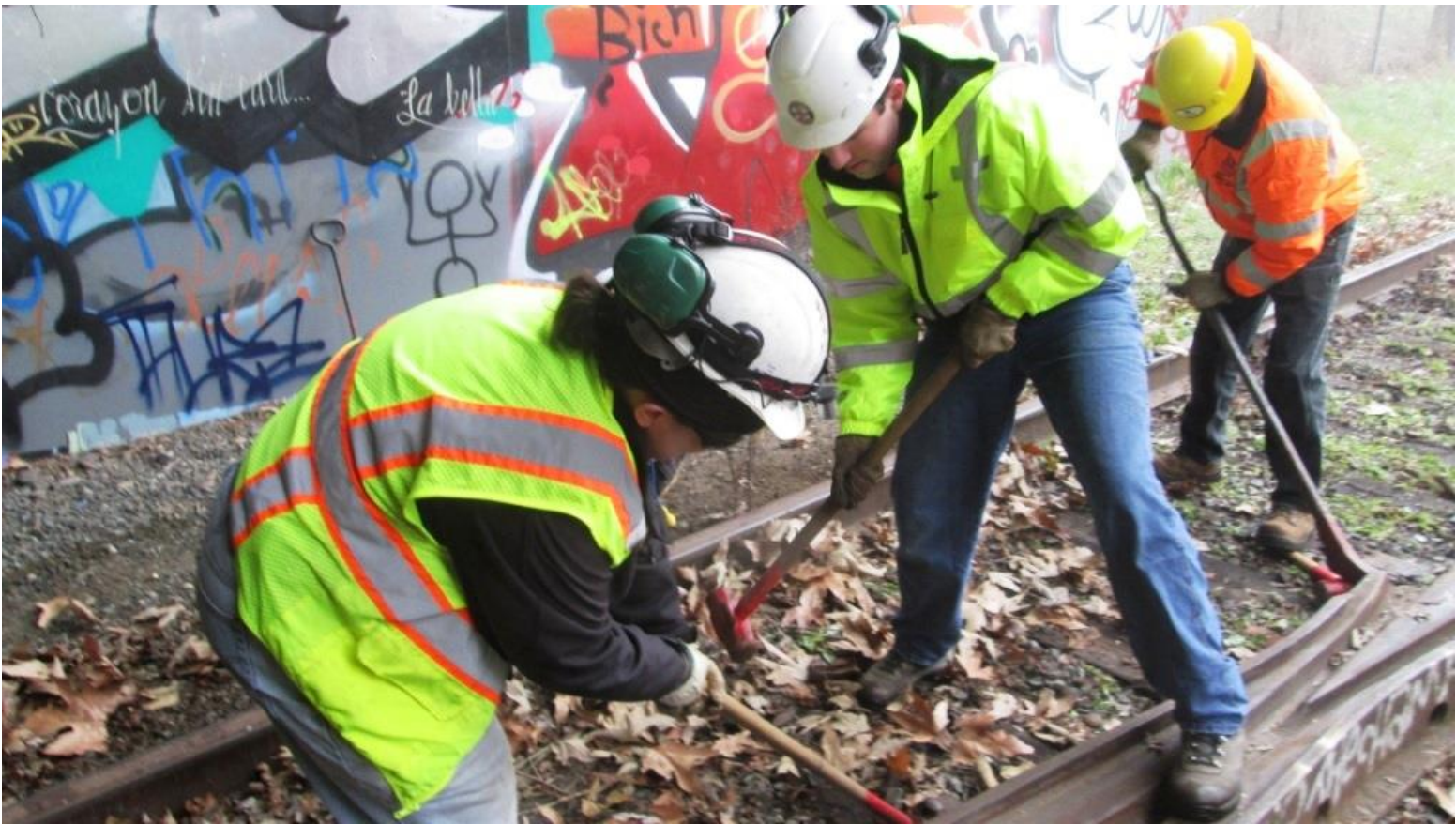
Now Heather and Weston use the spike-lifter to pry-up a spike
