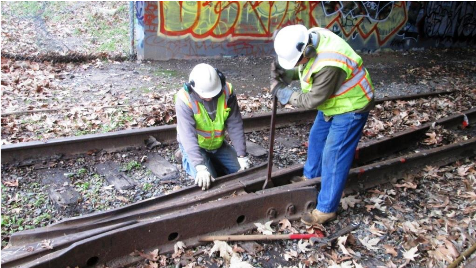
Steve and Clem start unbolting the frog from the rail
